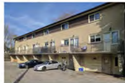
Nottingham Avenue, Kitchener 16 Unit Townhouse Complex
